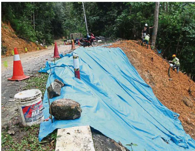
Tarp protecting a slope on the road leading to Air Itam Dam.
