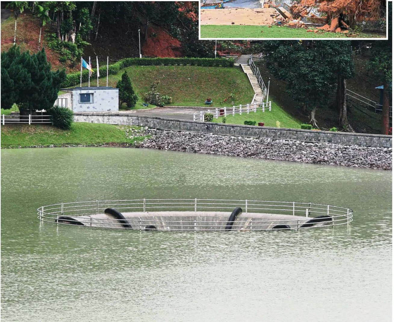
Full to the brim: The Air Itam Dam is filled to its full capacity after the downpour. (Top right) One of the landslides along the road leading to the dam. —LIM BENG TATT/The Star
